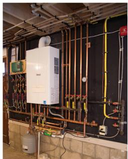
break rooms and employee washrooms; this can cut water heating energy use by 30% or more. Tank water heaters must use energy to make hot water available at all times.
